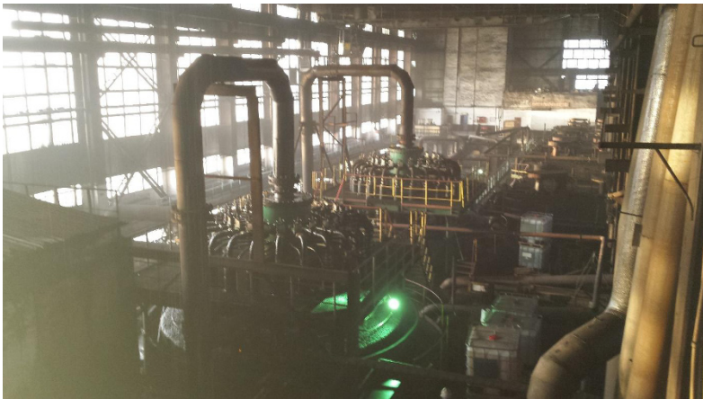
Figure 4 Jameson Cell Installation
