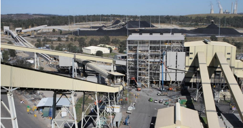
Figure 1 Ravensworth preparation plant and product stockpiles
