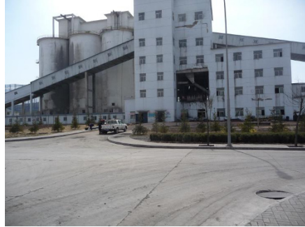
Picture 2: Shenhua Lijiahao CPP installation opening
