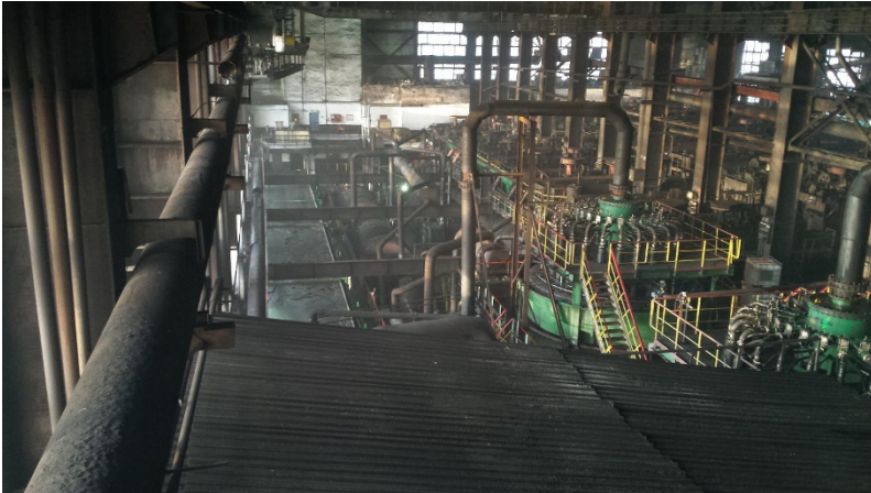
Figure 3 Jameson Cell and Delkor Filter Installation
