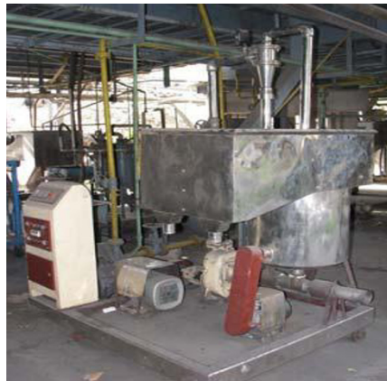
Figure-1: H. M. Cyclone Test Rig
