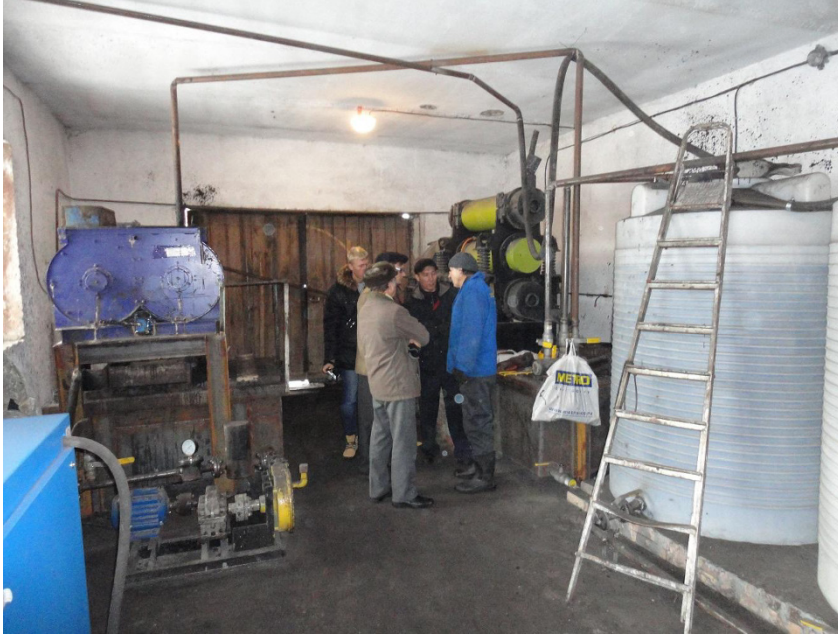
Figure 3 – General view of semi-industrial installation for CWF preparation and burning
