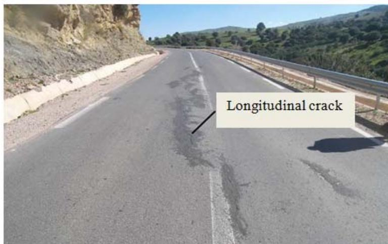
**Fig.1.** Embankment crack (February 2011) (DTP Guelma)
