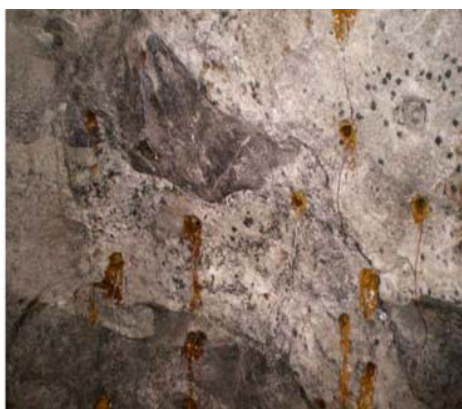
Figure 5. Charging of bulk Ukrainit-PP-2 EE with the help of ZEP-10 charger: (a) and (b) are charging process and the process termination respectively (general view)
