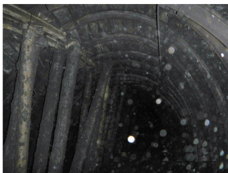
Fig. 2.6. The state of the 590 belt entry at a distance of at least 30 m (PK11) behind the 590 longwall face
