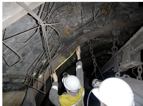
Fig. 2.4. The state of the 590 belt entry in the “window” area of the 590 longwall face
