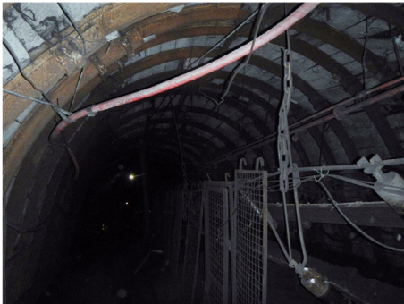
Fig. 2.3. Fragment of the 590 belt entry in the area from PK0 to PK4
