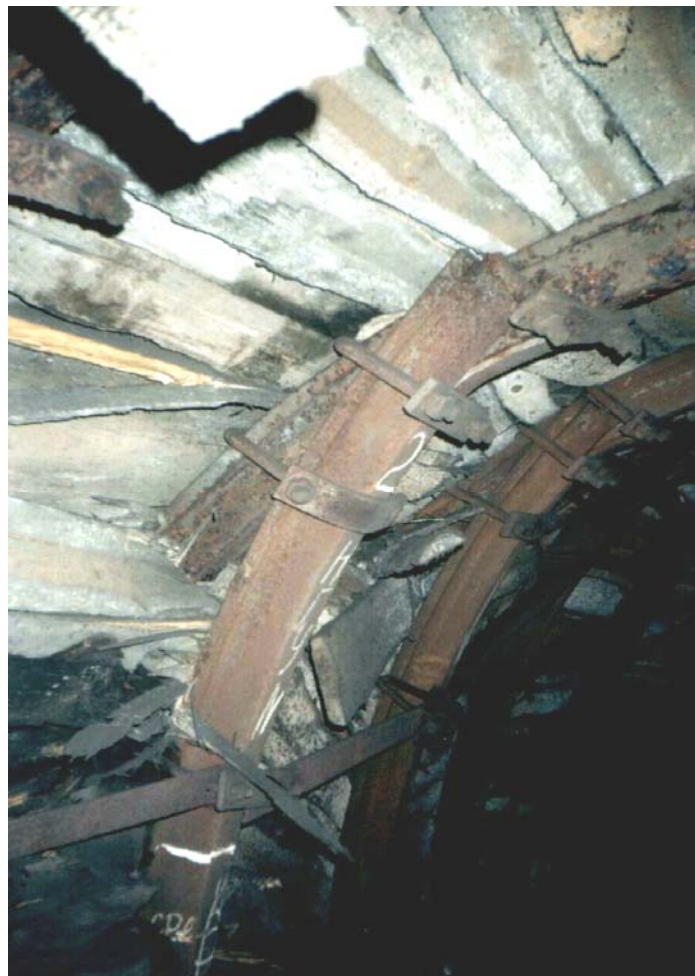
Fig. 3.17 Deformations of boundary entry 719 support: a) from worked-out area; b) from pillar
