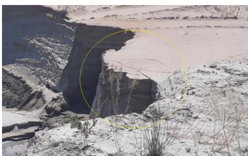
Figure 11. Deep crack in the III rd step of the North Peșteana open-pit
