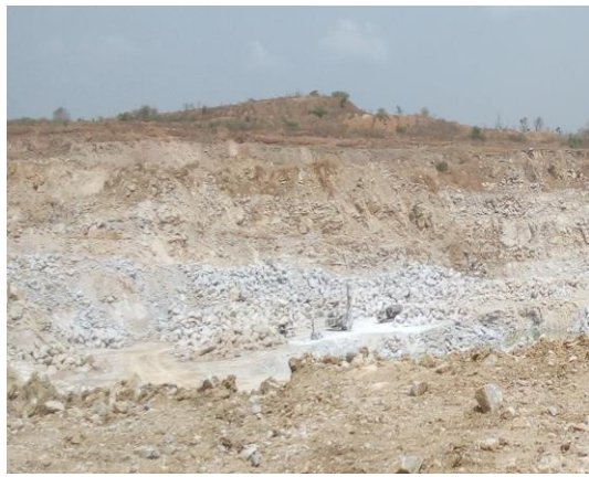
Figure 2. Obajana Quarry Site after Blasting (Pit 1)
