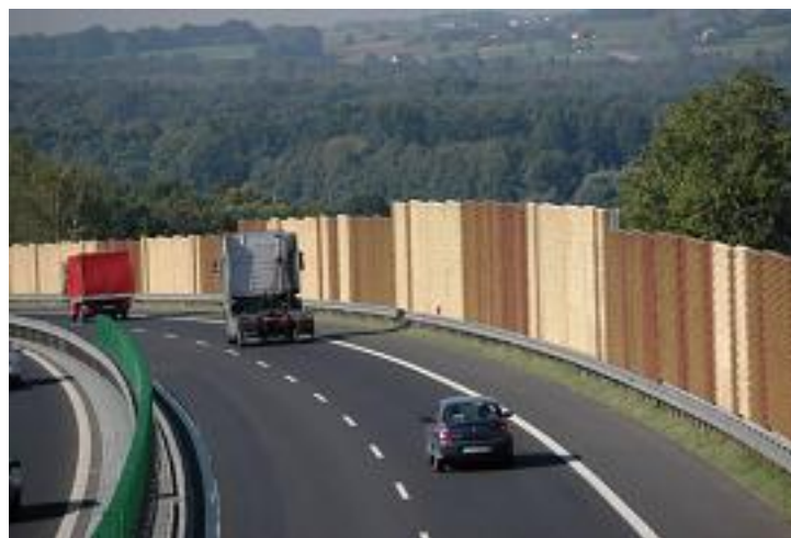
Fig. 2. Sawdust concrete noise abatement walls
