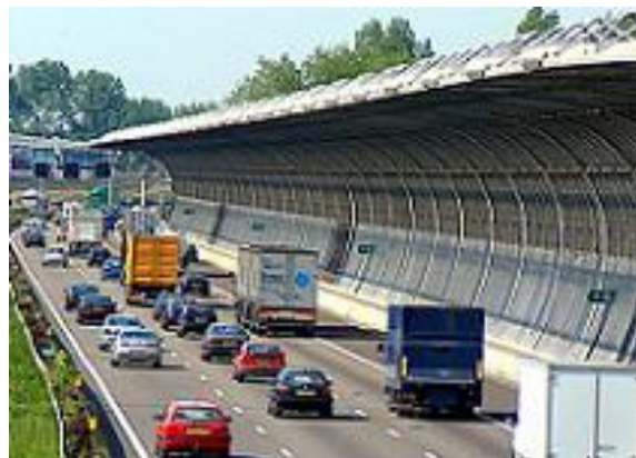
Fig. 3. Acoustic covering – a tall curved shield
