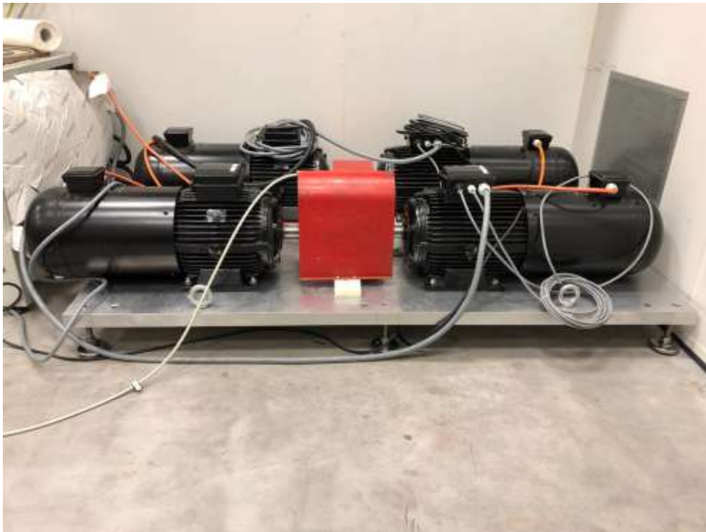
Figure 4.3 Installed red protective cover
