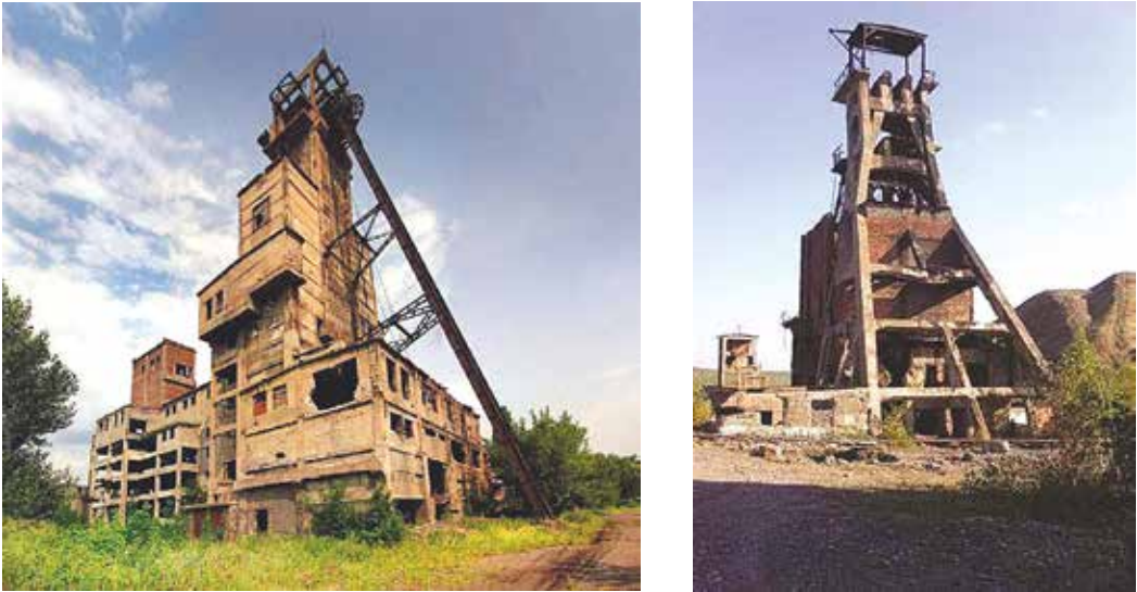
Fig. 6.17. Dilapidated buildings remaining on the abandoned mines
