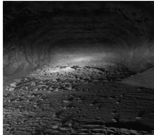
Figure 11 – Blast results with Riomax XE ordinary explosive type
