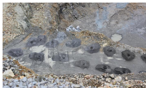
Figure 6. Boreholes in the experimental area of blasting operations
