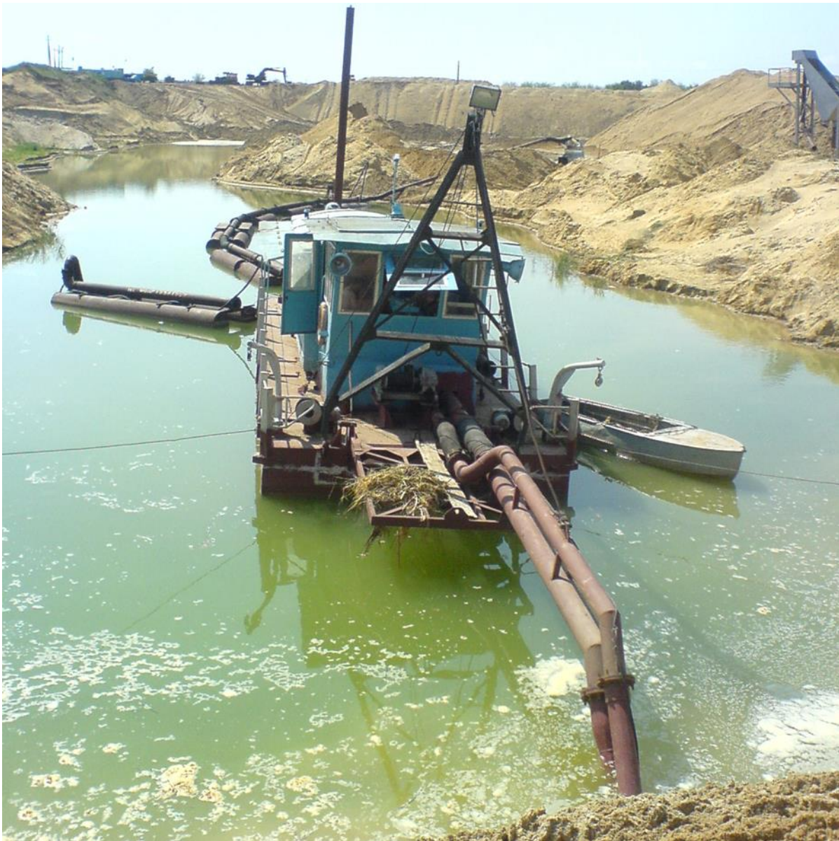
Fig. 4. The jet pump dredger JPD 300-120 in the face
