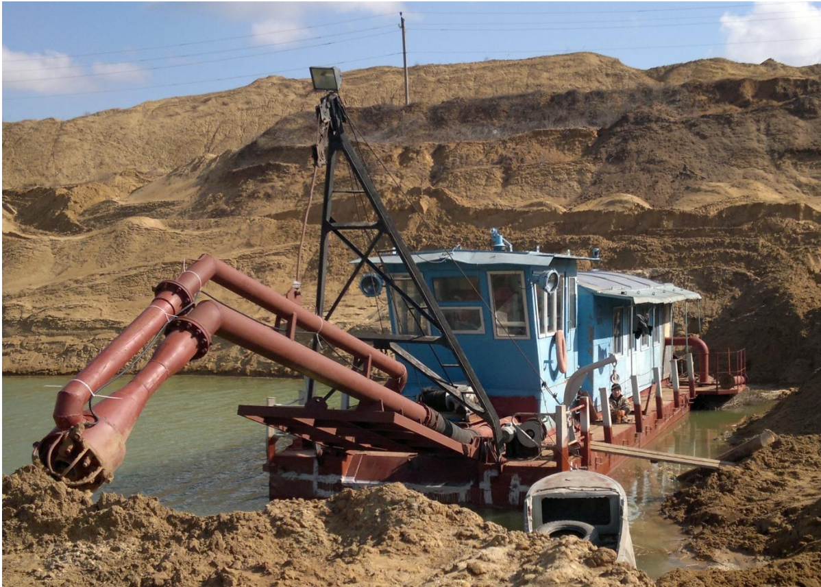
Fig. 3. Installation of equipment of the jet pump dredger JPD 300-120
