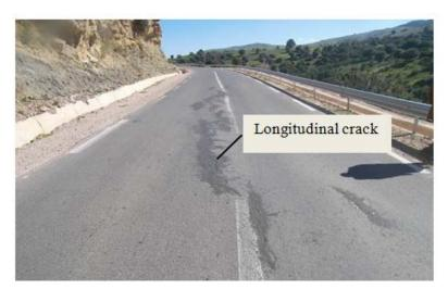
Fig.1. Embankment crack (February 2011) (DTP Guelma)
