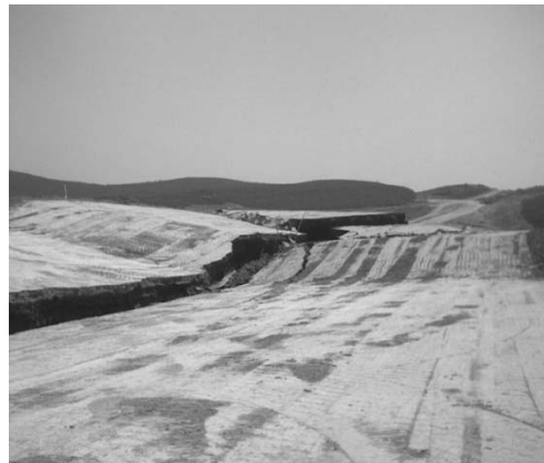
Fig. 11 Final Deformation of embankment.
