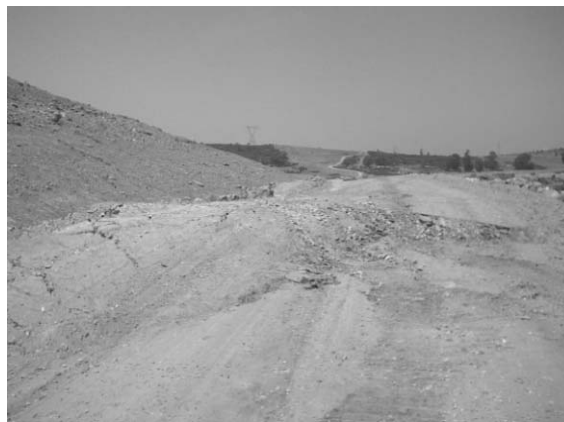
Fig. 7 Heave up on the embankment's foot to 15m high.
