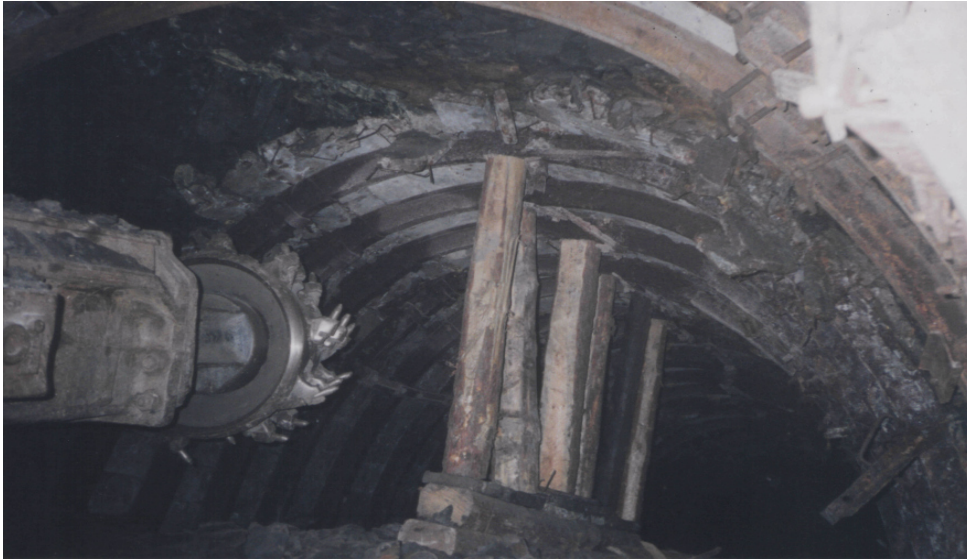
Fig. 4.21. Retimbering of boundary entry 115 with floor rock extraction (1.0 to 1.2 m) with the help of mining machine
