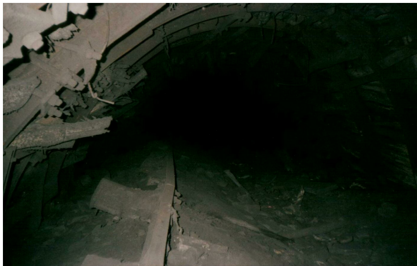
Fig. 4.20. Boundary entry 115 after retimbering: a) retimbering stope; b) 100m behind the longwall; and c) 250 m behind the longwall
