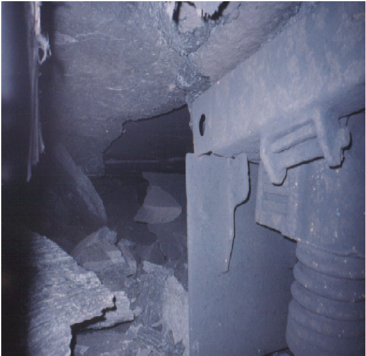
Fig. 4.9. Nature of roof rock hanging within worked-out area of C_6^1 seam
