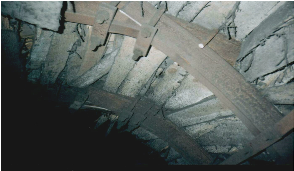
Fig. 4.19. Typical damage of arch support: a) from rock mass, b) and c) from worked-out area
