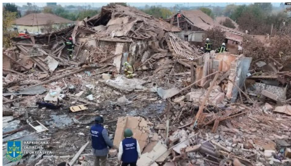
Fig.3. – Completely destroyed buildings
