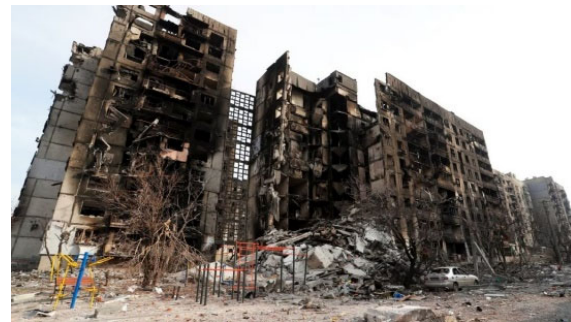
Fig.4. – Partially destroyed buildings
