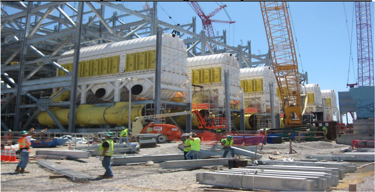
Fig. 3. Installation of boiling layer dryers HDC 9250 on thermal power stations IGCC (the USA, state Mississippi)
