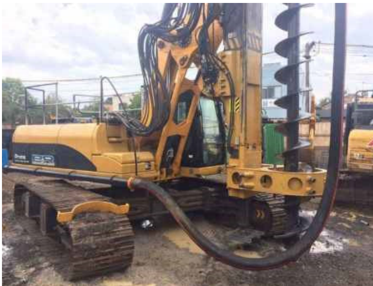
Figure 4.4 – Pile boring equipment
