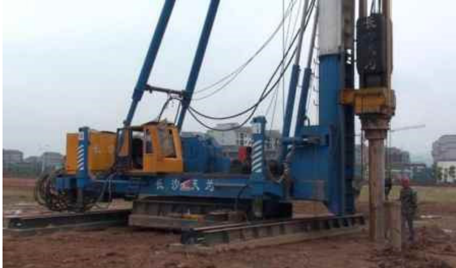
Figure 4.5 – Pile boring equipment
