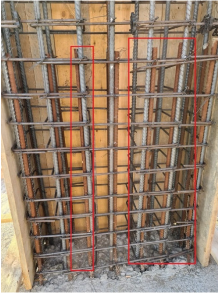
Figure 3.16- Connecting the steel link with a length of 1 meter
