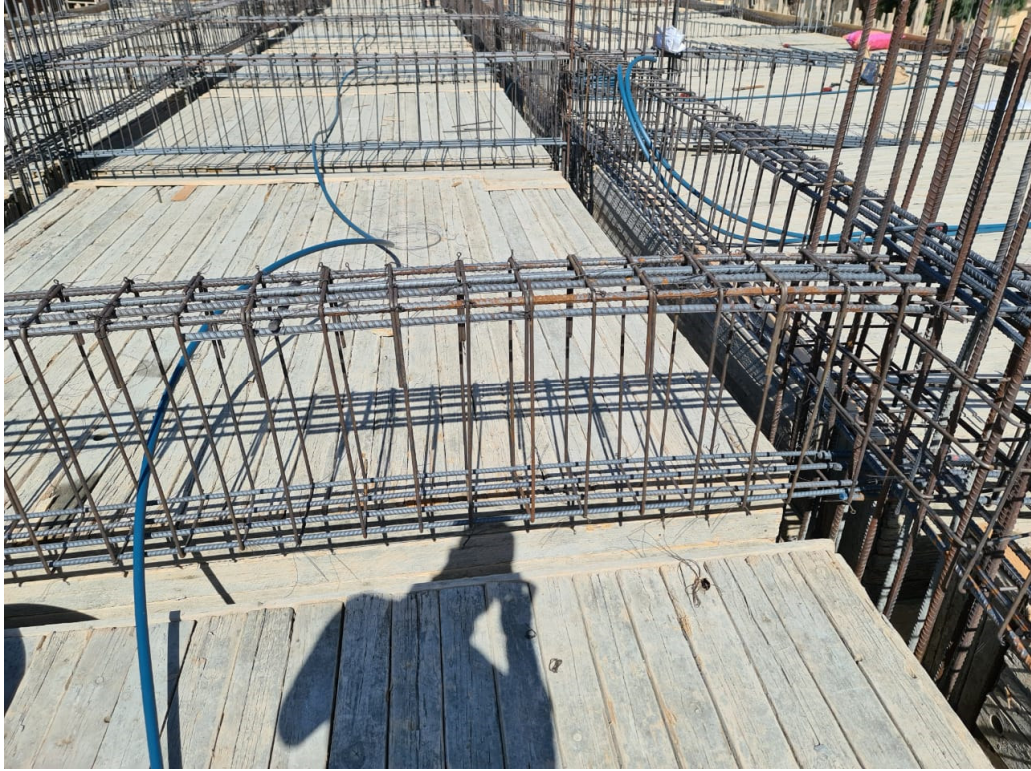
Figure 3.9- beam reinforced cages
