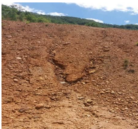
Figure 1. The first landfill
