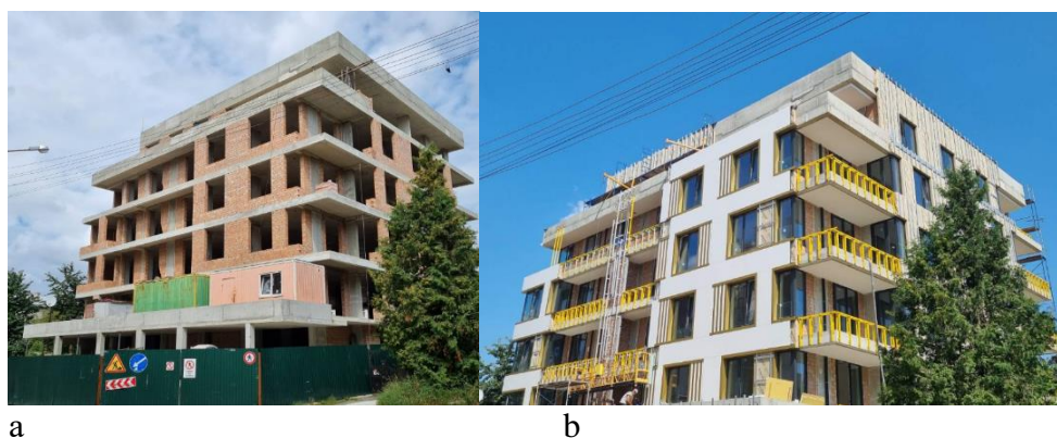
Figure 4 – a – Photo of the residential complex in 2022, b – Photo of the partially adorned building with facade, window, and door structures in 2023
